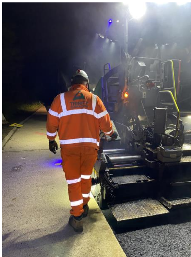
New asphalt surface being applied on the westbound carriageway
