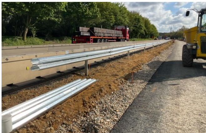
Above: New safety barrier installation on the westbound carriageway
