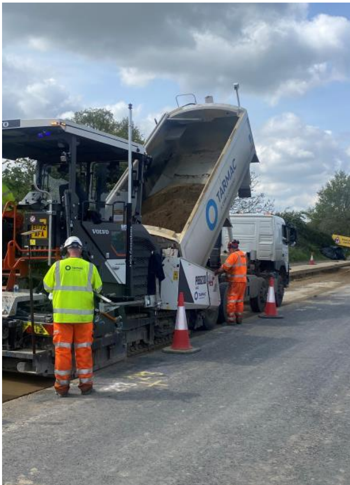
Above: westbound carriageway base foundation layer work completed this month.
